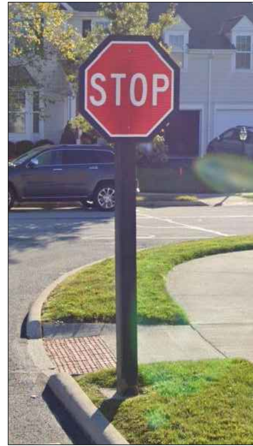
Typical Street Regulatory and Street Name Sign Signs per City Standard Drawings NA-SNS-1.2,3 & 4. Painted Green PMS 5535 or similar.
