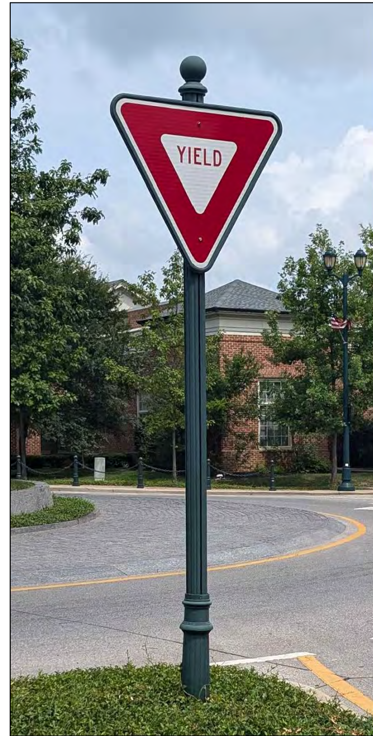
Typical Street Regulatory and Warning Signs Signs per City Standard Drawings NA-SNS-7,8 & 9. Painted Green PMS 5535 or similar.
