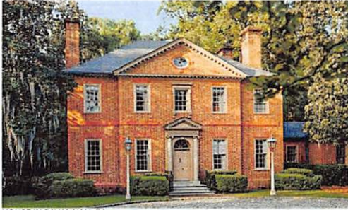
HOUSE IN SAVANNAH, GA.
